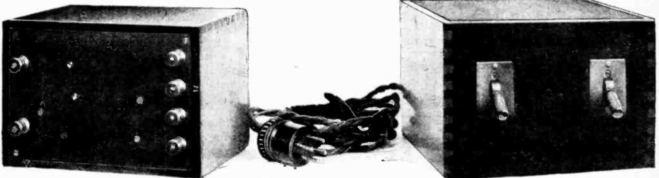
The relay unit (left) which is installed near the receiver, and (right) the control unit and adaptor for connection to the loud-speaker extension leads.
